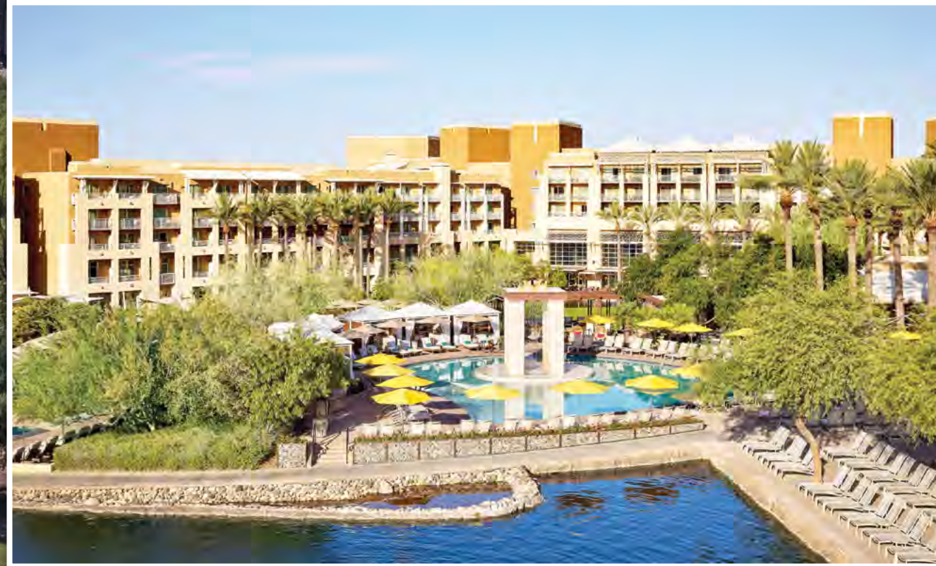
EXTERIOR POOL COMPLEX.
